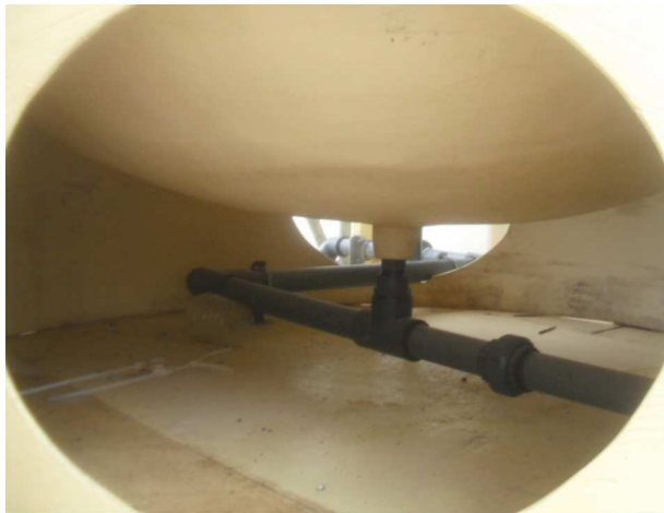
Figure 11 Scaffolding Works: Connection of the Tank Vents to the Scrubbing System
