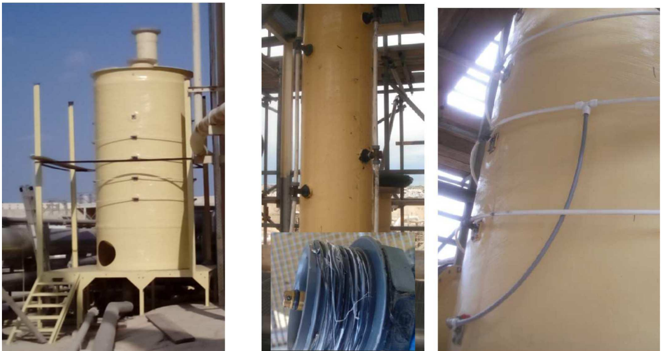
Fig 9 Installation of the Pre-Mix Chamber
