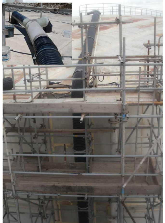
Figure 11 Scaffolding Works: Connection of the Tank Vents to the Scrubbing System
