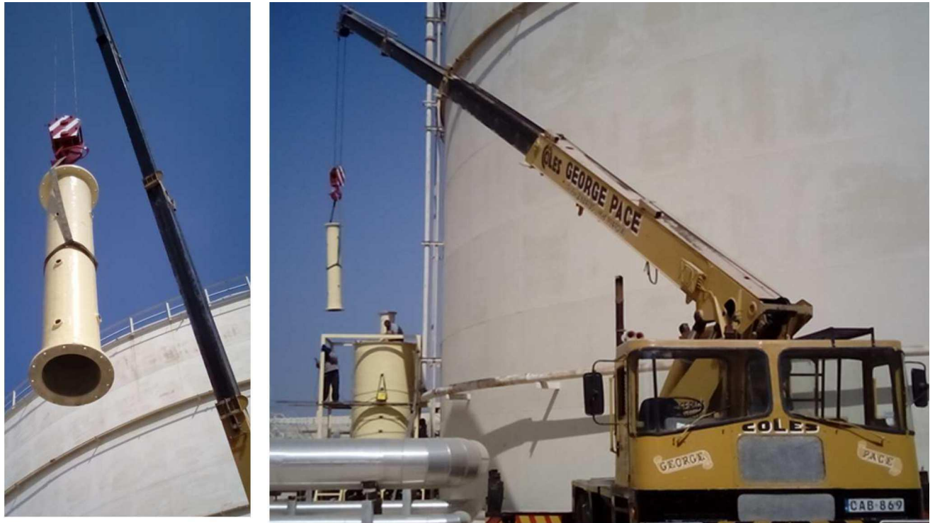
Fig 9 Installation of the Pre-Mix Chamber
